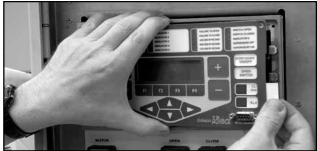
Figure 28. Removal of inserts from front operation panel of iDC switch control.
