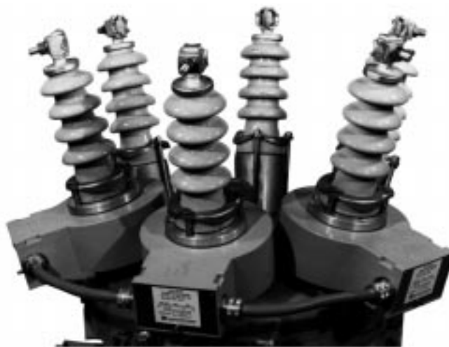
Figure 11. Bushing Current Transformer accessory mounted on recloser bushings. 82083KMA
