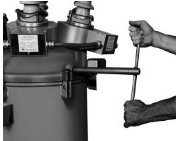
Figure 15. Using the manual closing tool to operate the recloser.
