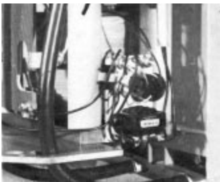
Figure 28. Type KFE low-voltage closing accessory, mounted on side of recloser mechanism.
