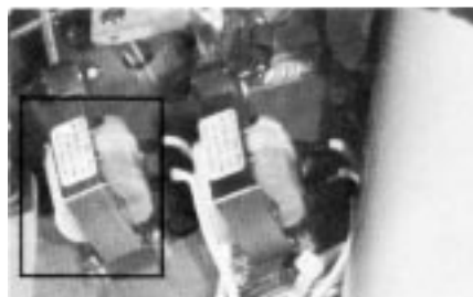
Figure 33. Remote-Lockout accessory KRK409F mounted on side of recloser mechanism. 82087KMA
