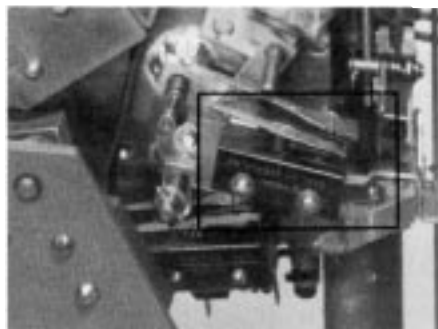
Figure 31. 82253KMA Lockout-Indicating Switch KRK412FA mounted on side of recloser mechanism.
