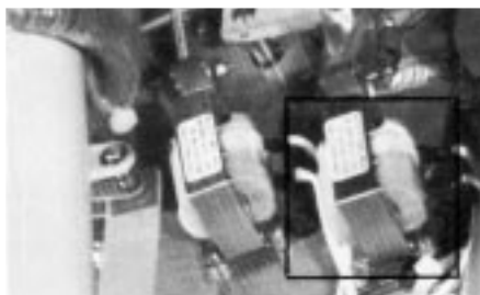
Figure 32. Remote-Trip accessory KRK410F mounted on side of recloser mechanism. 82087KMA
