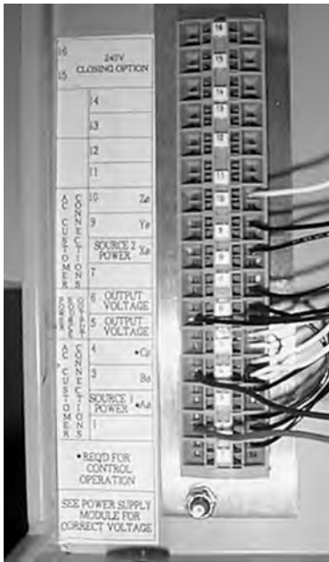
Figure 35. Terminal Connector Block TB1.
