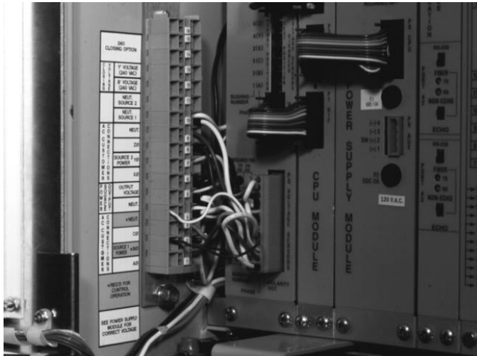
Figure 26. Terminal Connector Block TB1.
