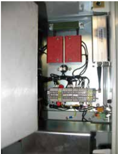
Figure 27. Radio mounting tray (example radio mounted) mounted on right-side interior cabinet wall.
