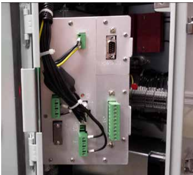
Figure 39. Side swing-panel view of SPEAR single-phase recloser control.
