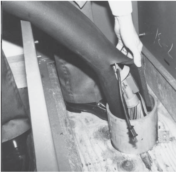
Figure 3. Completely cover thermostat with insulation.
