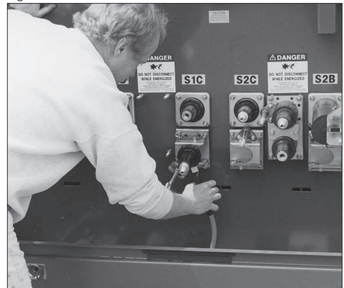
Figure 9. Installation of the standoff bushing.
