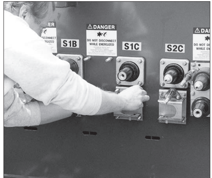
Figure 8. Installation of the parking stand.
