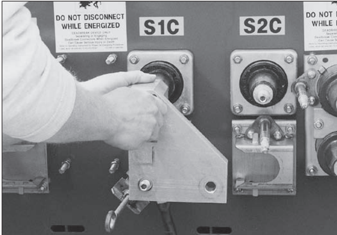
Figure 10. Using gauge to align parking stand.
