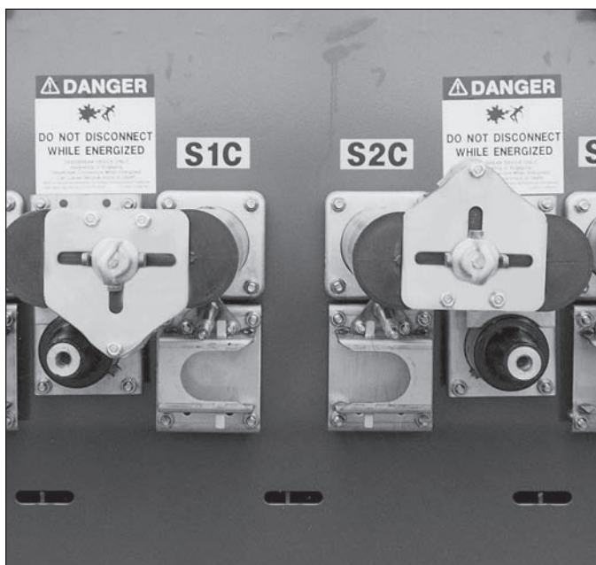
Figure 2. Left-hand and right-hand U-OP connector installations.
