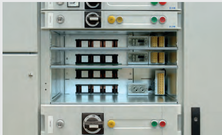
Compartments for withdrawable units including: IP2x shielding, outgoing and auxiliary contacts.
