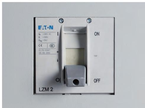
DIN control components and main switch with escutcheon interlock
