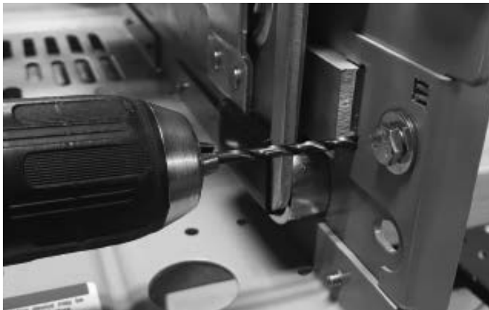
Figure 20. Drilling the bottom edge of template
