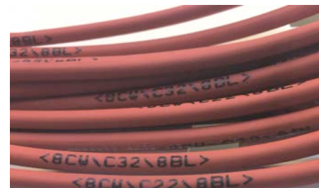
Control Wire Marking
