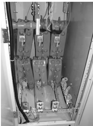
Grounding Balls and Covers
