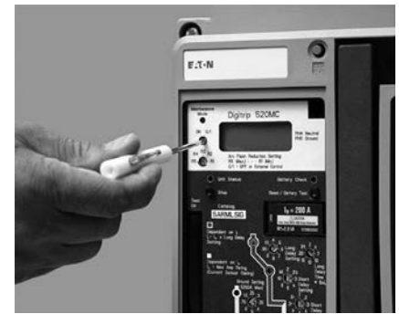
Arcflash Reduction Maintenance System
