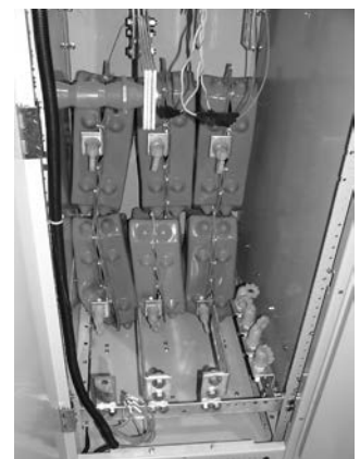
Grounding Balls and Covers
