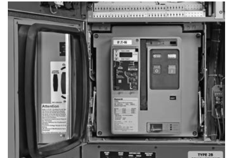
Bellows and Two-Point Door Latch
