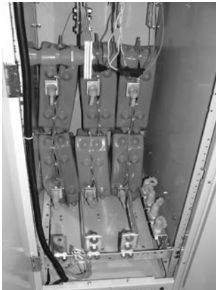
Grounding Balls and Covers
