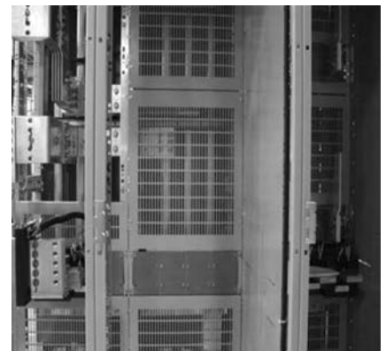
Optional Bus Compartment and Vertical Section Barriers
