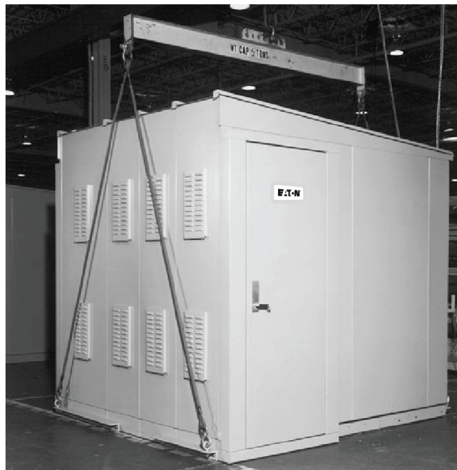
Figure 1. NEMA 3R Assembly Lifting Method.
