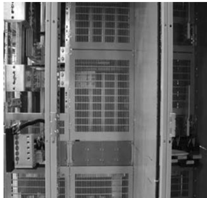
Optional Bus Compartment and Vertical Section Barriers
