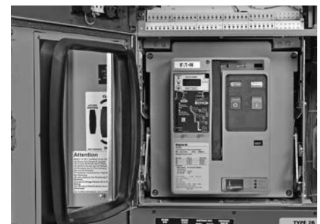
Bellows and Two-Point Door Latch
