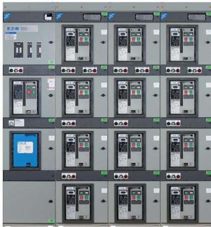
Arc Quenching Switchgear
