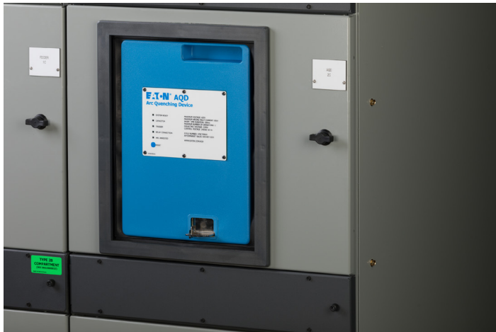
Figure 10. AQD in the connect position.
