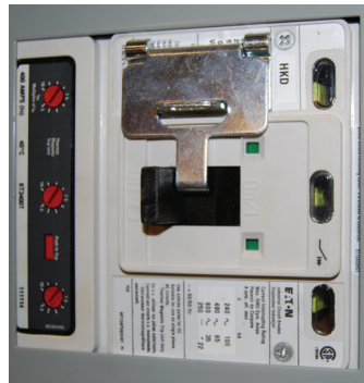
Breaker in OFF position with visual indicators through the VISA window.
