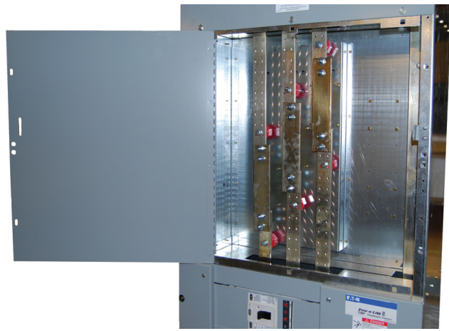
Utility compartment including three-phase bus, neutral bus, ground connection, and the locations of CTs and PTs.
