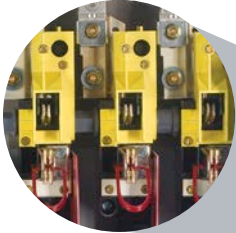
External window provides clear path to view the enhanced visible blade switching base
