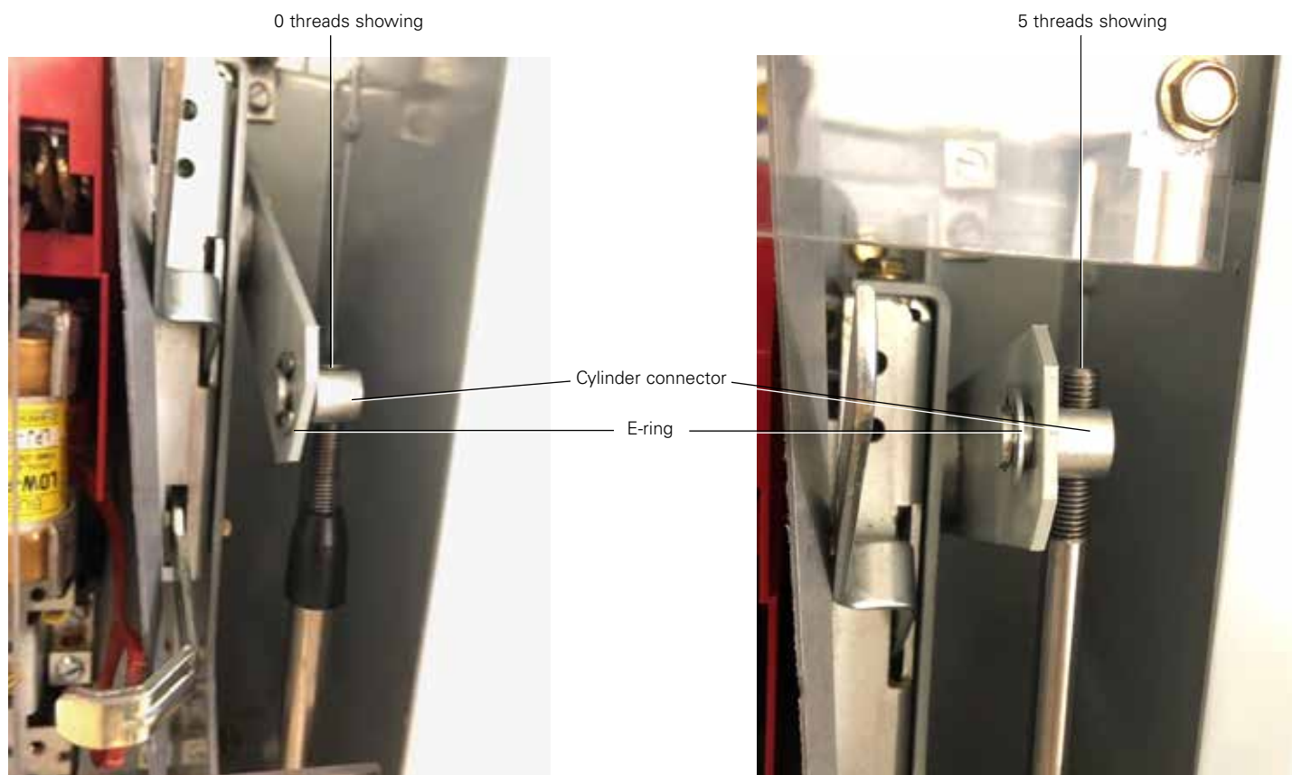
Figure 7. Location of cylinder connector threads and E-ring.
