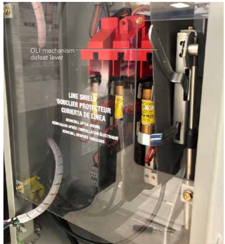
Figure 10. Lexan line shield and switch base.
