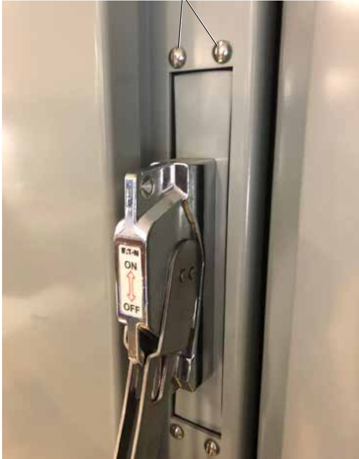
Figure 14. Handle mechanism and mounting hardware.
