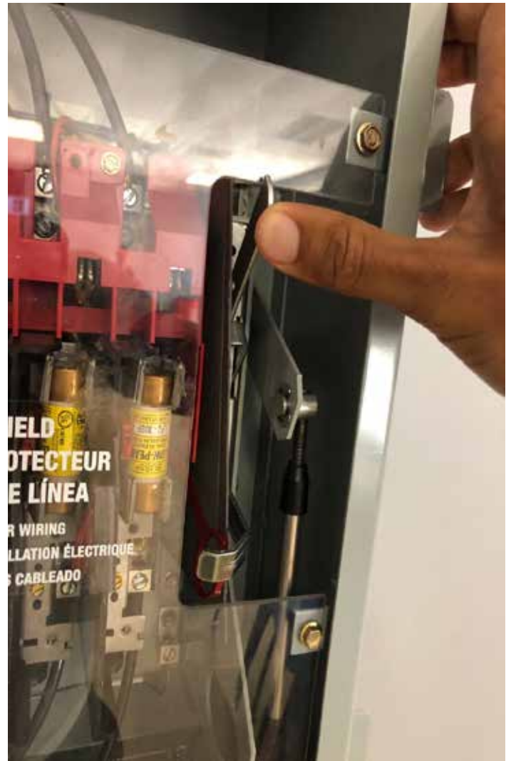
Figure 3. Defeat OLI door interlock.
