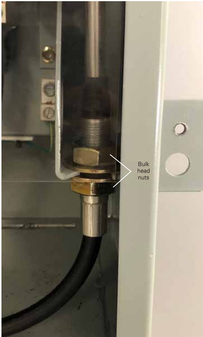
Figure 8. Correct placement of the bulk head nuts.
