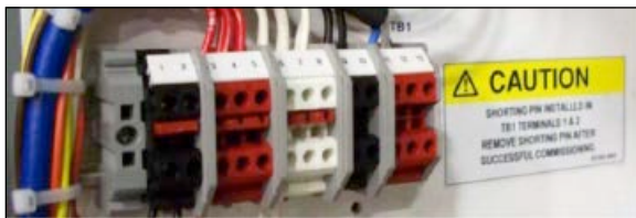
Figure 1. Terminal block TB1
