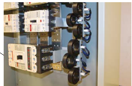
The current sensors are mounted on brackets in-line with the tenant breaker. Cable installation is made easy!
