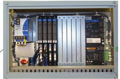
Current sensors are connected to the meter. This will eliminate timely installation cost.
