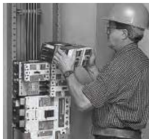
Panelboard Installation
