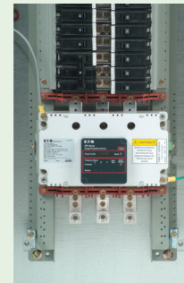
In this installation, the SPD Series is mounted directly to the panelboard's bus bars. This type of installation will provide the best possible surge protection by minimizing the connected lead length.
