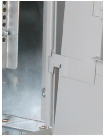
Photo 3. Trim Hanger Inserted into Box Flange
