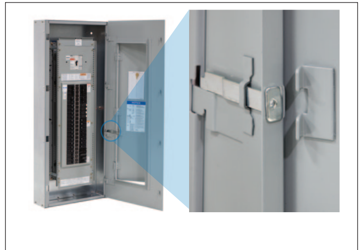
Figure 2. Trim Installed with Door Open and Anti-Lift Slide Bracket
