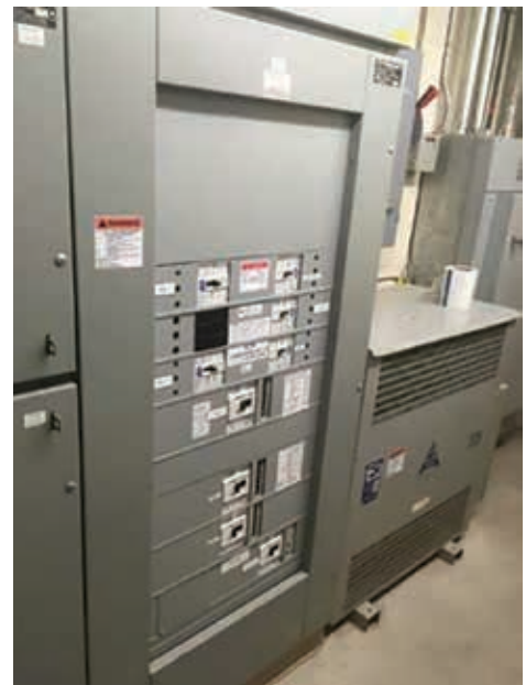
PRL 4RX Interior reduces installation time by using an existing enclosure with adjustable sliding mechanism
