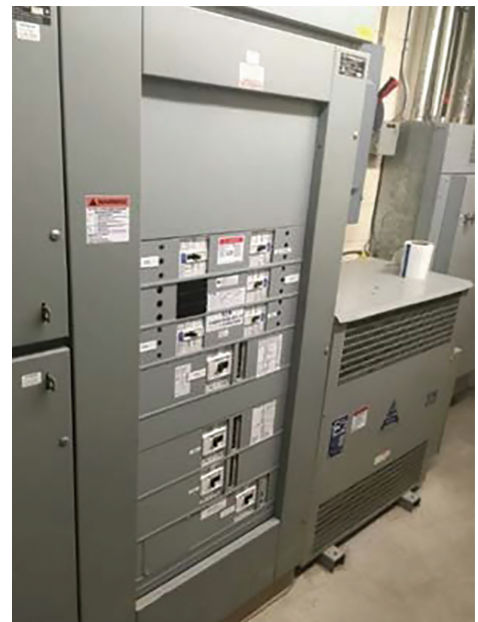
PRL 4R Interior reduces installation time by using an existing enclosure with adjustable sliding mechanism
