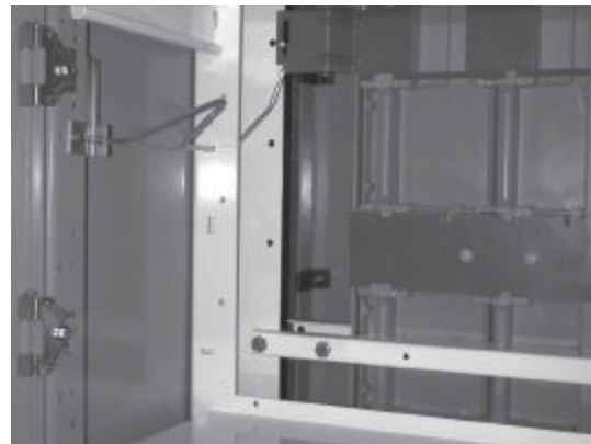
Figure 34. Shutter arm linkage
