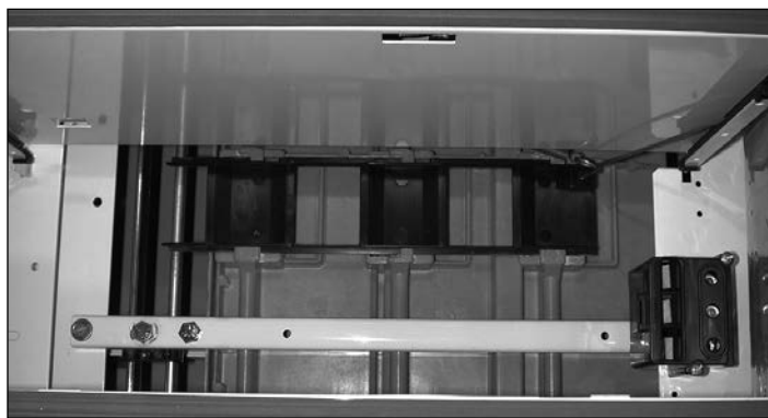
Figure 35. Shutter arm linkage
