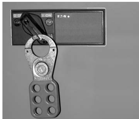
Figure 40. Correct application of scissors lock
