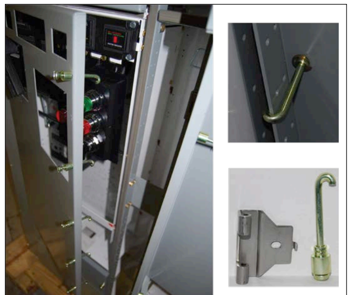
Figure 54. MCC unit and vertical wireway door latches and hinges
