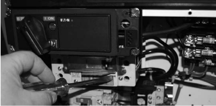
Figure 27. HMCP magnetic adjustment
