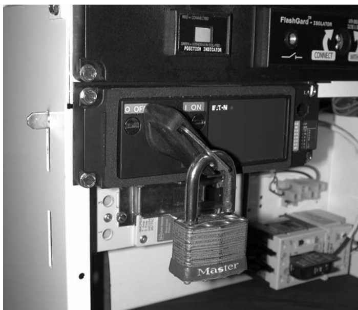
Figure 39. Locking out a disconnect
