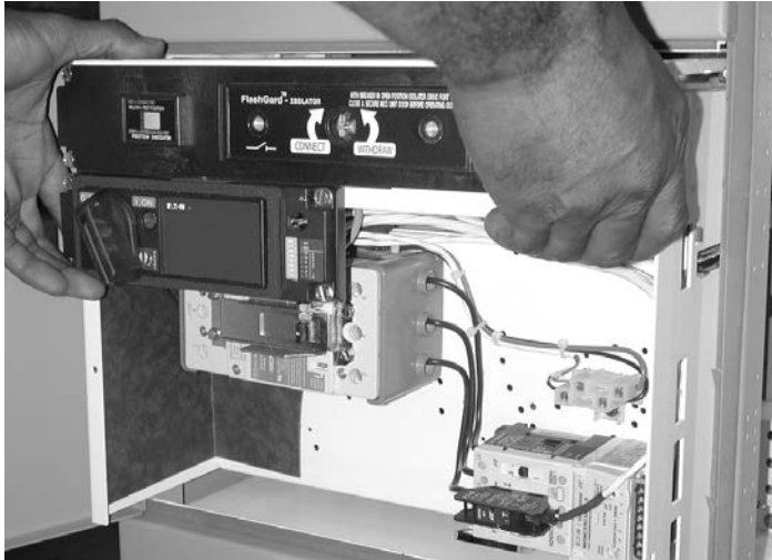
Figure 37. Withdrawing a unit
