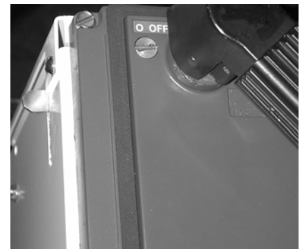
Unit Insertion Interlock
