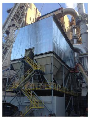
Fig. 4 New baghouse structure installed at the existing cement plant
