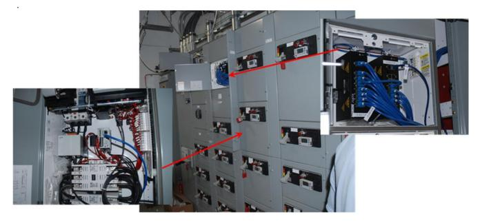
Fig. 6 Installed motor control center showing a starter unit at right and home-run connection to Ethernet switches at left
