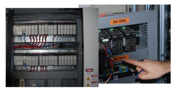
Fig. 7 At left, programmable logic controller panel with EthernetIP communication cards and input/output cards to support local field devices. At right, beginning and end of the network ring connection to the MCC
