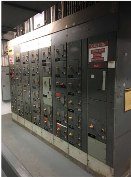
Fig. 6 Existing 45-year-old LV motor control center (left) and supplier proposed layout of replacement assembly (right)
