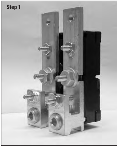
Step 1 Test Block in normal operation. All screw terminals are in the closed position and tightened to the required torque specification.
