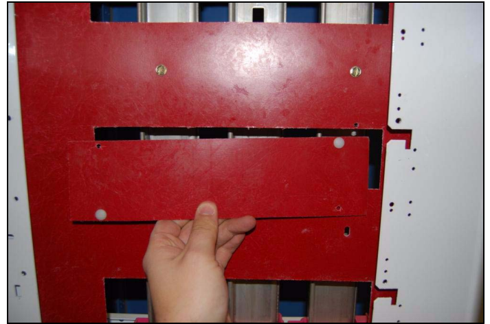
Figure 21. Shows the Installation of an Isolation Barrier Opening - Cover, Covers Are Provided with Upgrade Kit (99-5713-2).
