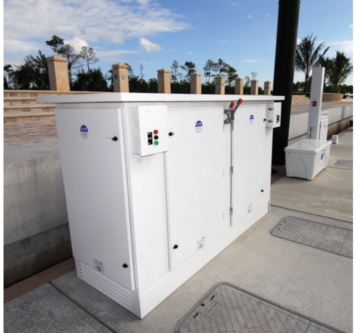
Above: Dual Panel Substation
