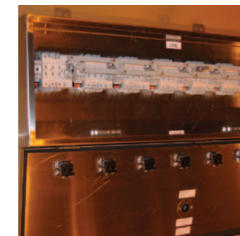
Disconnecting Multiple Loads Simultaneously
