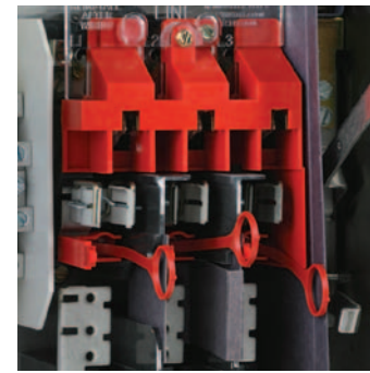
Factory-Installed Fuse Pullers
