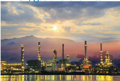
Oil, gas and chemical
