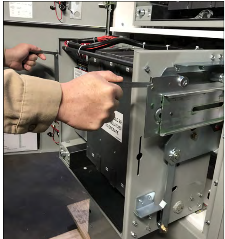
Figure 32. Pushing in Contactor.
