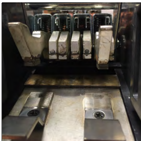
Figure 35. Contacts Behind ARC Chutes.
