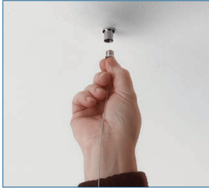
2. Thread drop wire through lower half of suspension boss and screw into the upper section on the mounting surface
