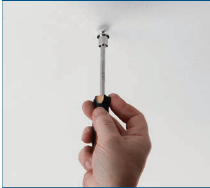
1. Secure suspension boss to the mounting surface
