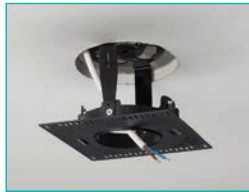
2. Cut aperture, insert first fix bezel and feed cable
