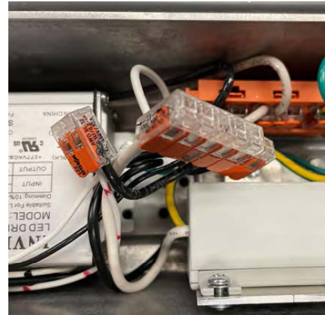
Figure 2: Surge Module Input Wiring Connections
