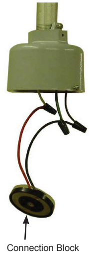
Figure 6 - Wiring Connections
