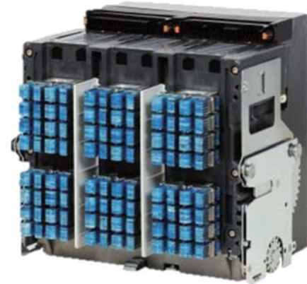
Breaker rear side (withdrawable breaker)
