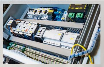
In the switch cabinet, the easy821 control relay, PKZ motor protectivecircuit-breakers and DIL contactors ensure safe, reliable operation.
