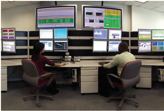
A three-tiered slatwall design allows for high-density monitor placement with clean sight lines to plasmas.
