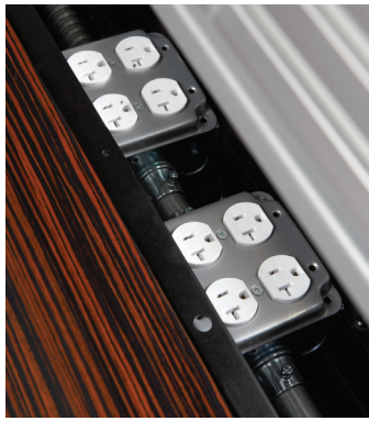
High-density technology requirements necessitated a modified core featuring hardwired power quad boxes; covered by removable brush strip panels.
